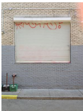
Window with the shelter closed 閘門關上後的大窗
